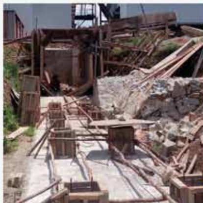
PEKERJAAN BOX CULVERT & STEAM PIPE SUPPORT
